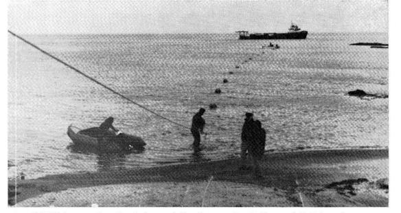
CABLE from underwater instrumentation to recording trailer park is being strung by a crew from the "Sea Tender." The instruments recorded shock wave in the sea around the island resulting from the Milrow detonation.
